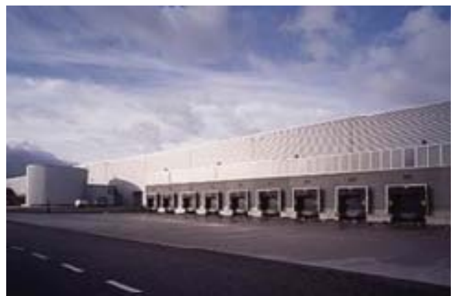
Figure 8: Sony Supply Chain Solutions (Europe)'s Tilburg Logistics Centre
